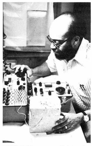
ADRIAN JONES measures residual stress in a tuff sample from the Nevada Test Site. Strain in the sample was measured, then overcored (circular cuts in the center of the block) and measured again by strain gages tied to the surface of the rock.
